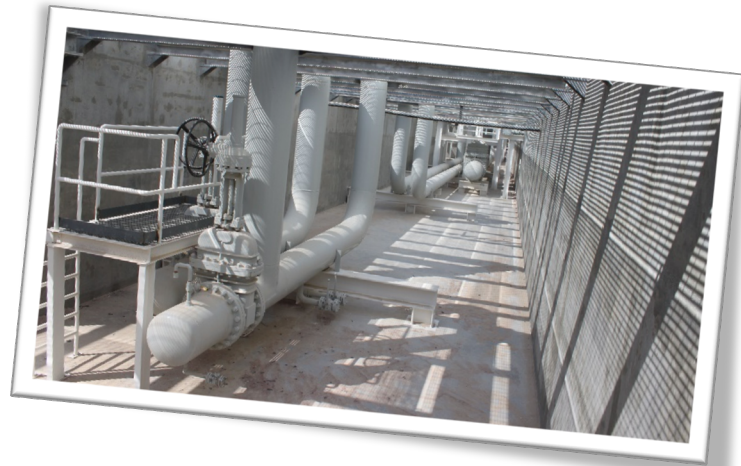
Fuel Delivery and Transmission Pipeline Systems and Associated Piping adjacent to a Jet A-1 fuel storage tank in a fuel farm facility
